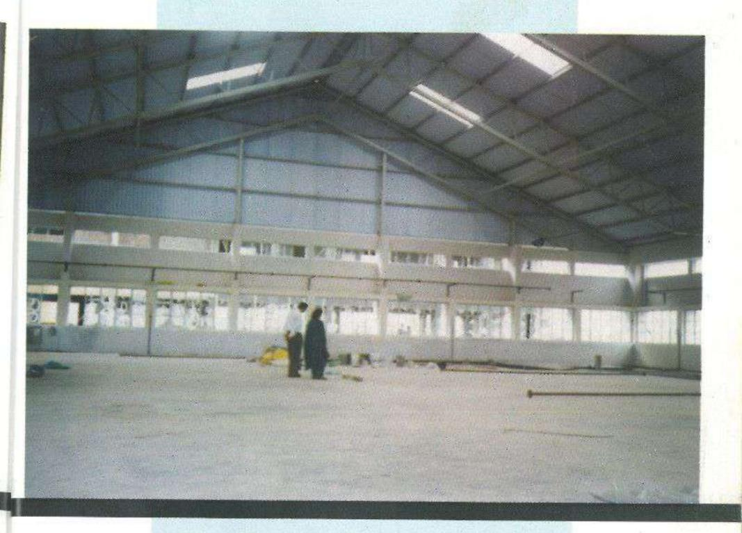
glass, use of water is intensively used in machine process. Surface gutters with m.s.grill to drain the fallen water are provided. As per machine layout size of machines, this gutter is provided only where there is use of water. An overlooking mezzanine is created at one end to overlook and supervise the machine operation. Here too some administration activities are carried out. An annex for the toilet block, compressor and generator is provided which solves the problem of segregating noise.
